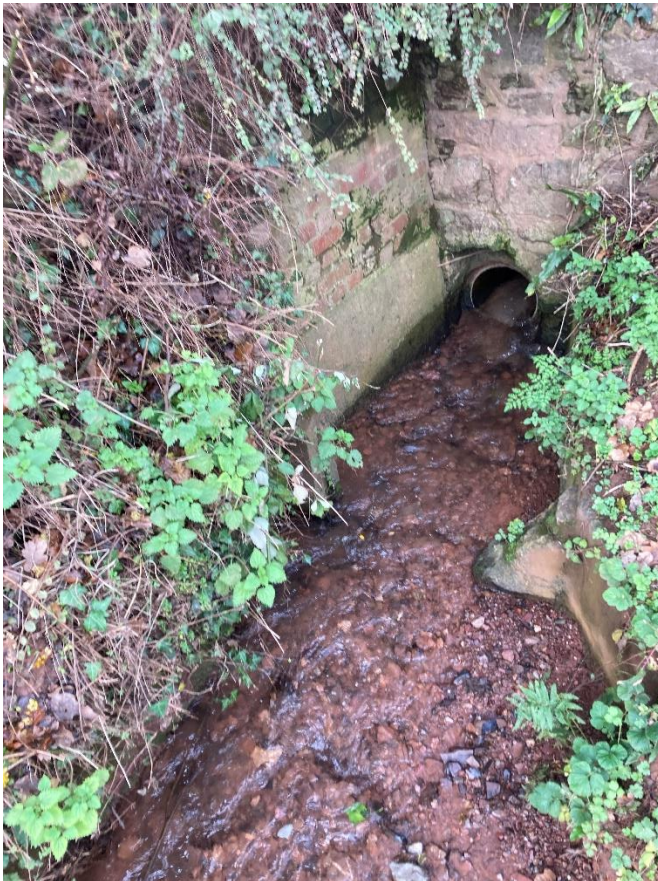
Figure 1- Culvert south of Ide
